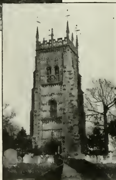
GREAT TOWER OF EVESHAM ABBEY (Actual Condition)
